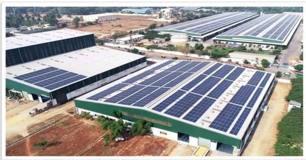
Figure 13. Solar photovoltaic (PV) system installations
