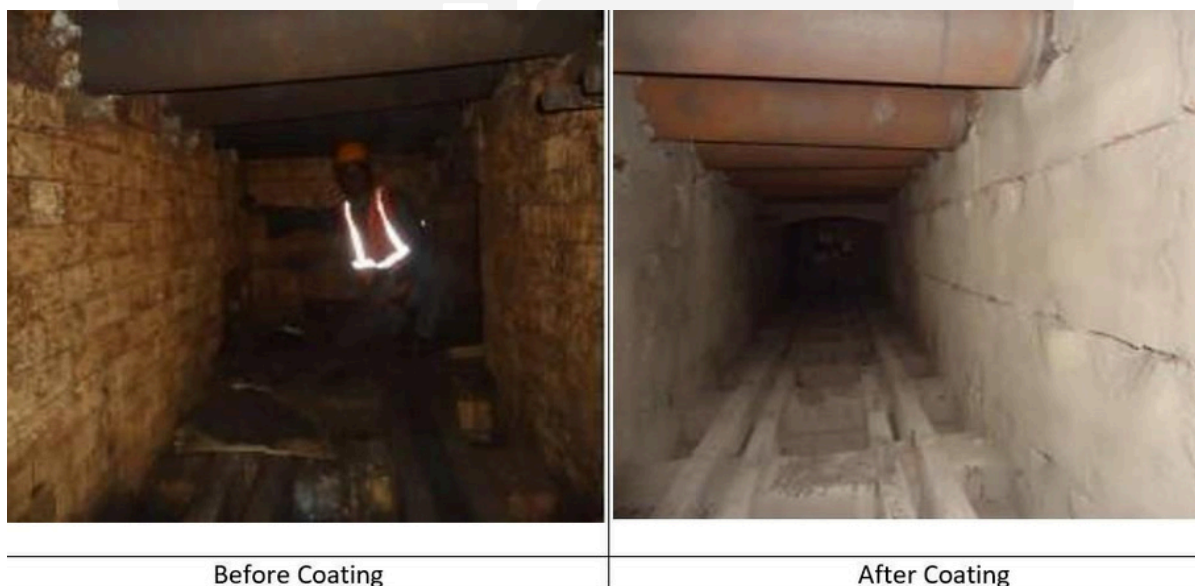
Figure 7. Thermo Ceramic Coating-Before and After application.
